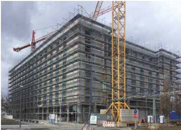
ABOVE: Steady progress on the building site
